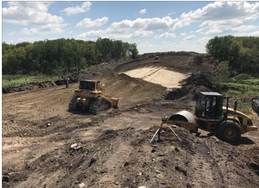
Water retention dam built close to Beulah, Manitoba, August 2017.
