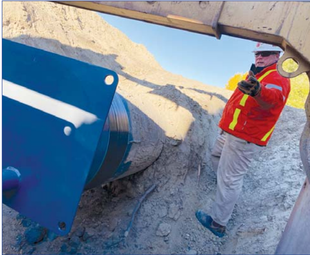
Left: Inspector Sandy Armstrong shows a section of pipe following installation of a steel cap. After the pipe segment is cut, a cap is fabricated onto the ends of the pipe and coated with epoxy. This permanently seals the pipeline at that location and backfill can then be completed.
