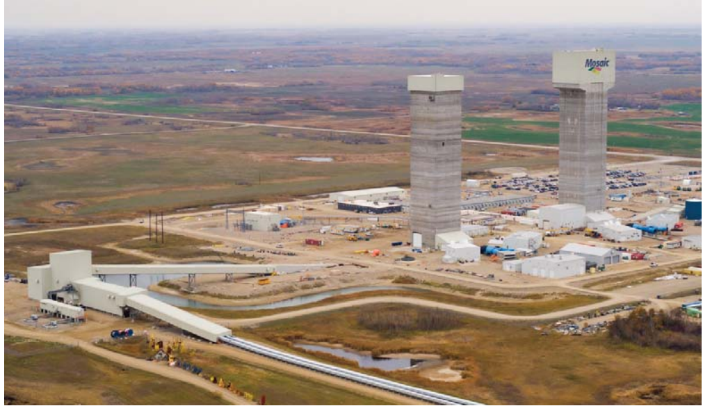
The K3 potash mine at Esterhazy. The south shaft headframe, at left, was completed this year. At the bottom of the photo the overland conveyors, which transport ore to the K1 and K2 mills, can be seen.
