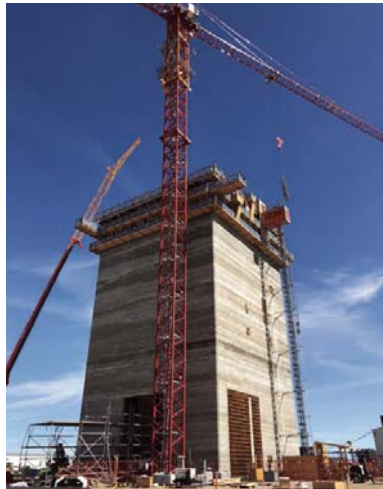
This photo shows the continuous pour on the south headframe at Mosaic K3 taking place, part of the $3 billion expansion of Mosaic Esterhazy's K3. The pour was completed on September 4.
