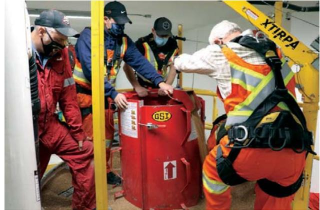
**Above left and right:** These photos show how to rescue someone using special equipment if they sink into the grain. Metal panels are pushed down around the person to create a tube and isolate them, above left. The grain is then augered out of the tube, right, and the person is lifted out once the level of grain in the tube is reduced.
