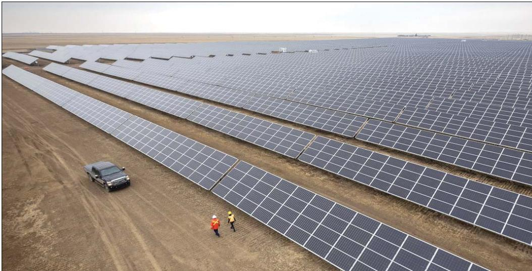
Enbridge's first solar self-power project in Canada between Lethbridge and Medicine Hat. Alberta Solar One, as it's known, supplies a portion of power to the Enbridge Mainline pipeline network, which includes the Line 3 replacement pipeline. The facility features 36,000 solar panels and has a capacity of 10.5 megawatts, equivalent to meeting the energy needs for about 3,000 homes and offsetting 12,000 tonnes of carbon annually.
