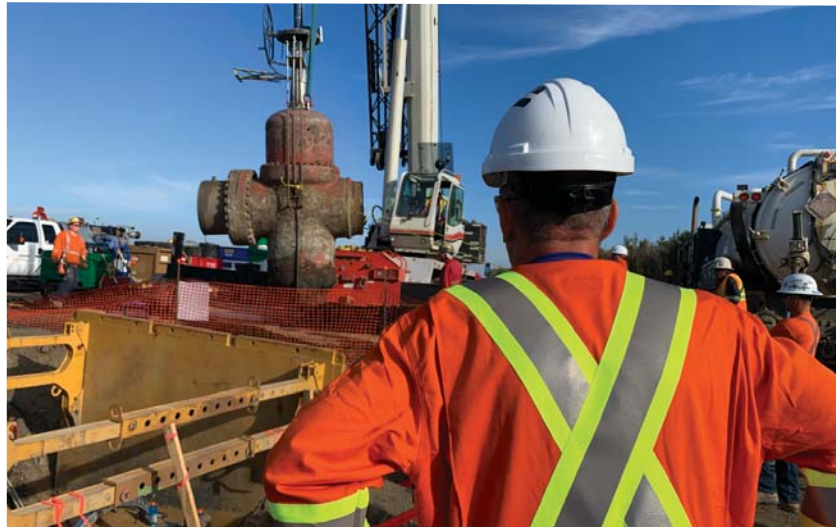
Contractors and Enbridge personnel remove a valve during Line 3 decommissioning near Morden, Manitoba. Small construction crews will be visible to the public doing similar work along the pipeline's right-of-way in southern Saskatchewan beginning in early June.
