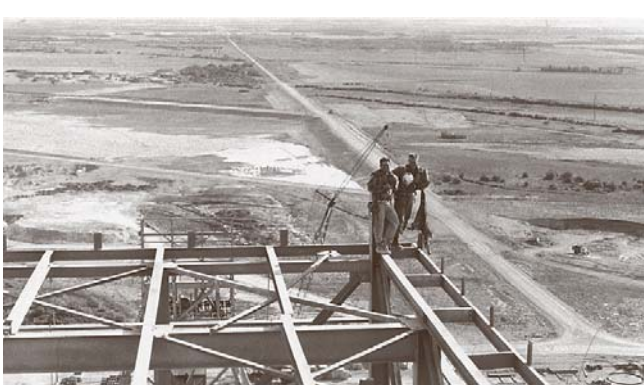
Above and right, construction on the headframes during initial construction of the Rocanville potash mine. Below, a new headframe under construction over top of one of the original headframes when the original service shaft was converted to a second production shaft, and a new service shaft was developed at Scissors Creek in 2011.
