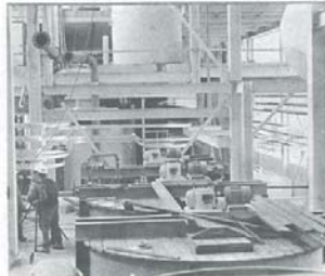
A portion of the re-agent mixing area at the refinery. At the extreme upper right can be seen a part of the dryer.
