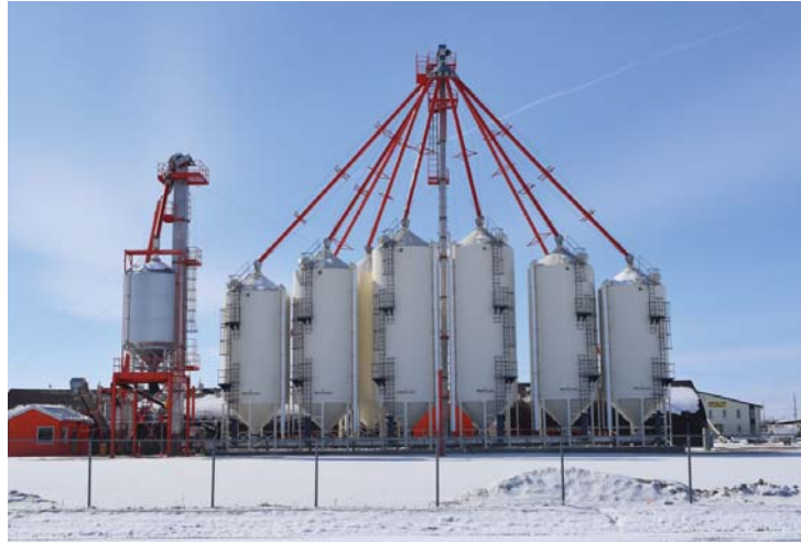
The new fertilizer blending facility at Sharpe's Soil Services in Moosomin will look similar to this but will be larger, with eight tanks on each side, not six.
