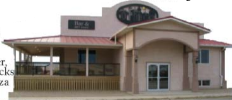
The Office Where You Don't Mind Putting In A Little Overtime!
