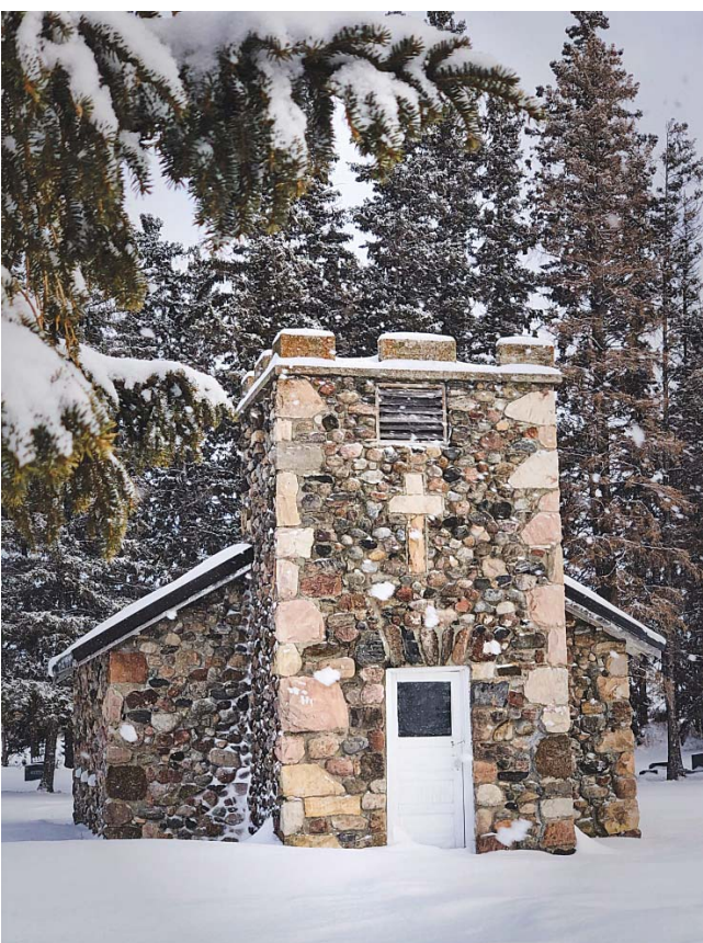
Above: St. Paul's Anglican Church in the RM of Wawken near Langbank. Built with fieldstone in 1938 by Charles Parker, a stonemason originally from Ontario.
