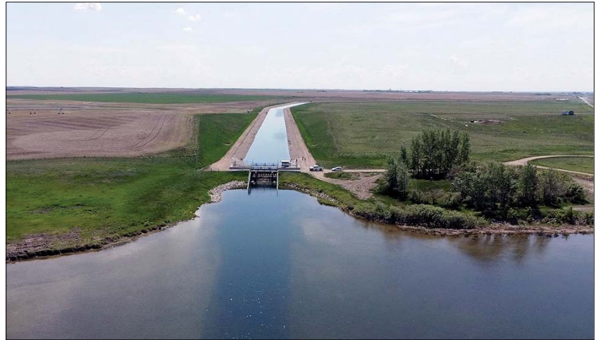
A canal connecting to the Broderick Reservoir, built in 1967, and located approximately 82 kilometres south of Saskatoon.
