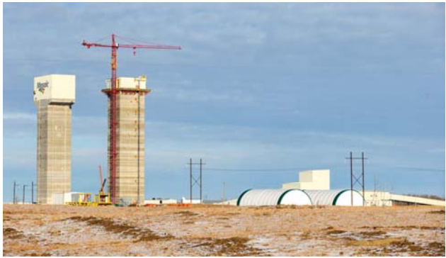
When the south shaft headframe is fully operational in March 2022, it will double the hoisting capacity at K3. Each shaft will have 36,000 tons per day hoisting capacity—for a total of 72,000 tons.
