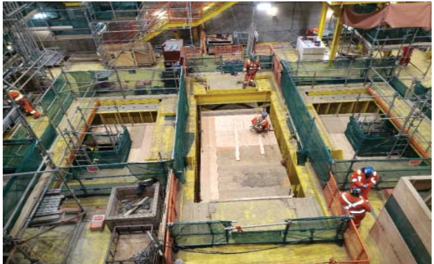
Construction activity on the Koepe hoist floor
