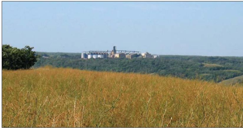
Bunge Harrowby – Canola crushing plant and refinery
