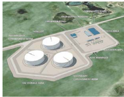
TransCanada's Energy East project would include a tank terminal at the Moosomin compressor station, including three 350,000 barrel tanks for a total capacity of 1,050,000 barrels of oil.
